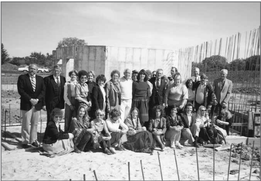
Construction starts with many problems ahead.
